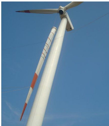
Fig 4. Straight Blade Erection
