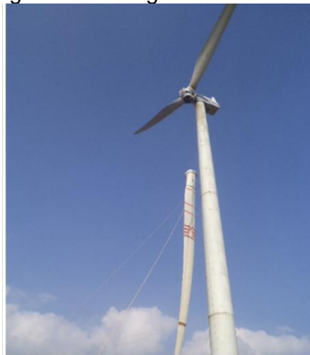
Figure 6. Pre-Bend Blade Erection
