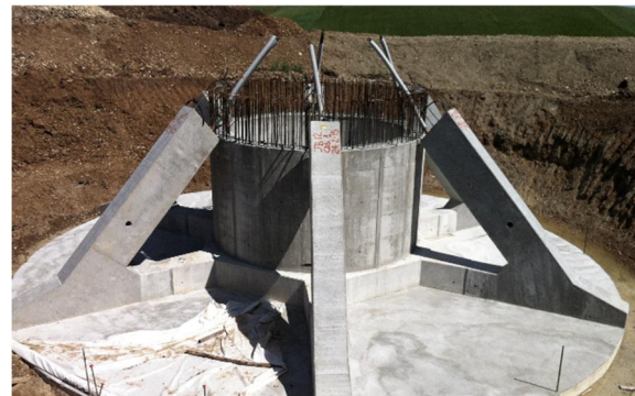
Figure 1 – General view of the precast braced foundation during construction works
