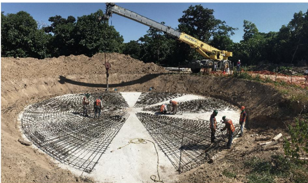
Figure 1 – General view of the precast braced foundation during construction works
